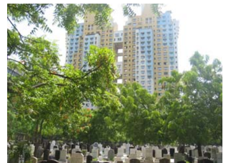
The multistoried building on the Worli cemetery premises (in the foreground)
